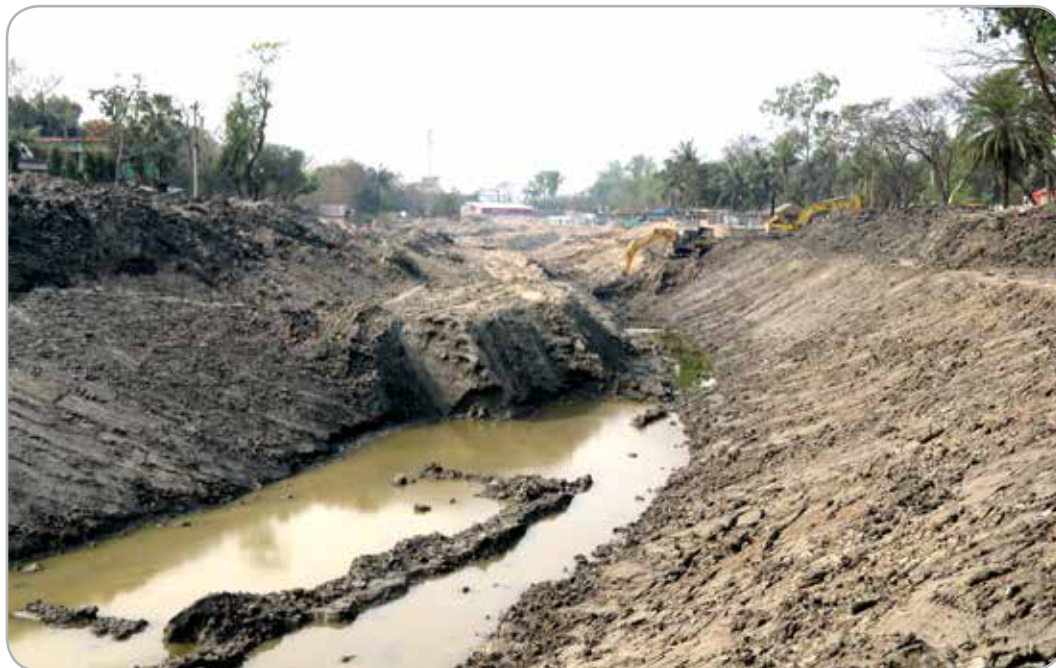
Excavation work in Bilgulli Canal at Satkhira.
